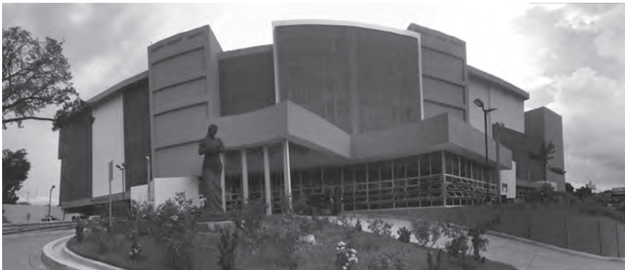
Image E1.2 New infrastructure of the National Women's Hospital in El Salvador (Boris Flores)
